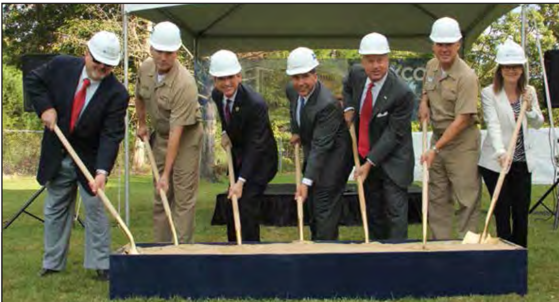
Wielding shovels in the Oct. 21 groundbreaking for the NEXCOM headquarters building expansion were (left to right) Randy Gibson, president, general contractors Whitesell-Green Inc.; Rear Adm. Ricky Williamson, USN, commander, Navy Region Mid-Atlantic; Congressman Scott Rigell, Representative of Virginia's 2nd District; Rear Adm. Robert J. Bianchi, SC, USN (Ret.), NEXCOM chief executive officer (CEO); William Sessoms, Virginia Beach Mayor; Capt. Kit Chope, USN, commanding officer, NAS Oceana, Va.; and Lisa Lingerfelt, project executive, DPR Construction.
