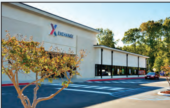
The renovated 65,000-square-foot Redstone Arsenal, Ala., Exchange recently underwent its first remodel in 14 years.
